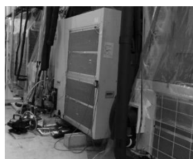
Fig. 6 CO 2 Cascade system
