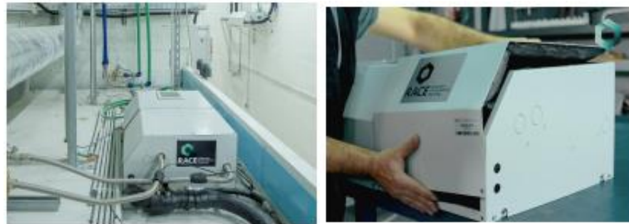
Fig. 3. Cooling boxes on the display cases
